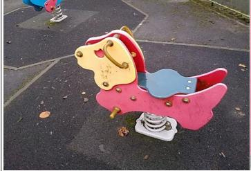
**Finding:** The end of footrests have a cross section of less than 15cm2 and fail to meet the requirements of BS EN 1176 Part 6
