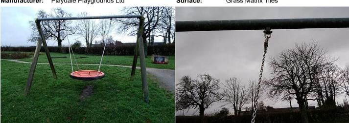
**Finding:** Swings of this design should have a secondary safety device fitted to prevent collapse of the seat in the event of a joint failure to meet the requirements of BS EN 1176 Part 2
