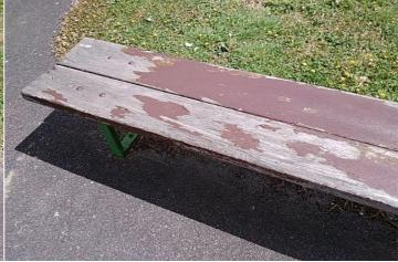
Finding: Flaking coating may create splinter / abrasion hazards
