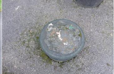
Finding: There is some evidence of fire damage to the item Action: Replace or repair as required
