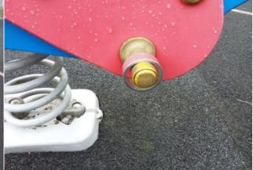
**Finding:** The end of handgrips and/or footrests have a cross **Action:** Monitor - No remedial work recommended section of less than 15cm2 and fail to meet the requirements of BS EN 1176 Part 6; this is however, a relatively low risk failure and no remedial action is recommended
