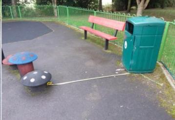
**Finding:** The bin forms a hard object within the falling space **Action:** Monitor - No remedial work recommended of the equipment in contravention of the requirements of BS EN 1176 Part 1
