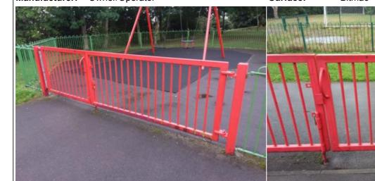
**Finding:** The gate is closing too quickly (less than 4 seconds)
