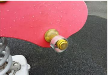
**Finding:** The end of handgrips and/or footrests have a cross **Action:** Monitor - No remedial work recommended section of less than 15cm2 and fail to meet the requirements of BS EN 1176 Part 6; this is however, a relatively low risk failure and no remedial action is recommended
