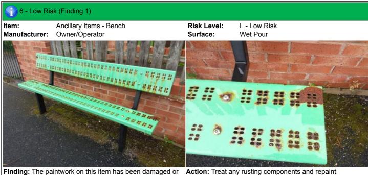
worn exposing the metal underneath which is rusting
