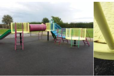
**Finding:** The paintwork on this item has been damaged or worn exposing the metal underneath which is rusting
