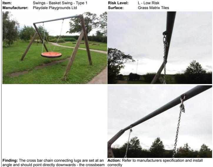
has been installed incorrectly
