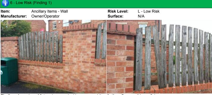
**Finding:** A number of fixings have worked loose around the **Action:** Secure all loose fixings fencing
