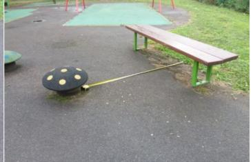
**Finding:** The bench forms a hard object within the falling space of the equipment in contravention of the requirements of BS EN 1176 Part 1
