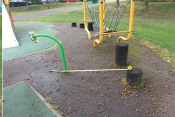
Finding: The talk tube forms a hard object within the falling Action: Monitor - No remedial work recommended space of the equipment in contravention of the requirements of BS EN 1176 Part 1
