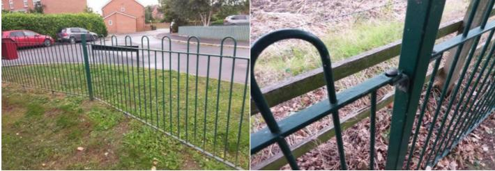
**Finding:** A number of fixings have worked loose around the **Action:** Secure all loose fixings fencing
